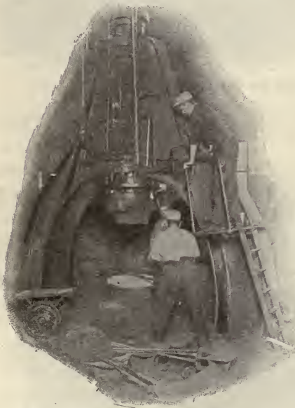
This Steam Hammer strikes a blow equal to 2½ tons.
