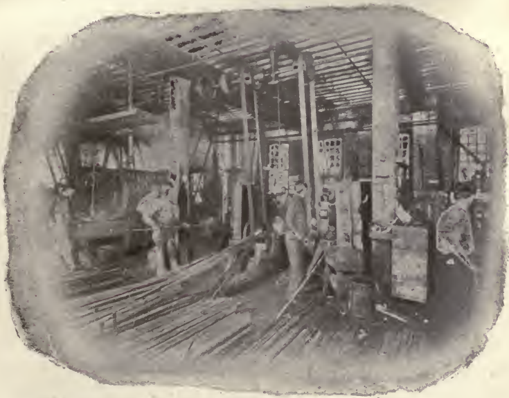
Steel Room, Cutting to Multiples.
