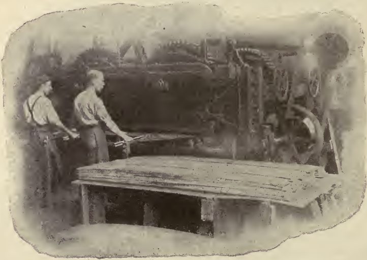
Cutting to shape.
