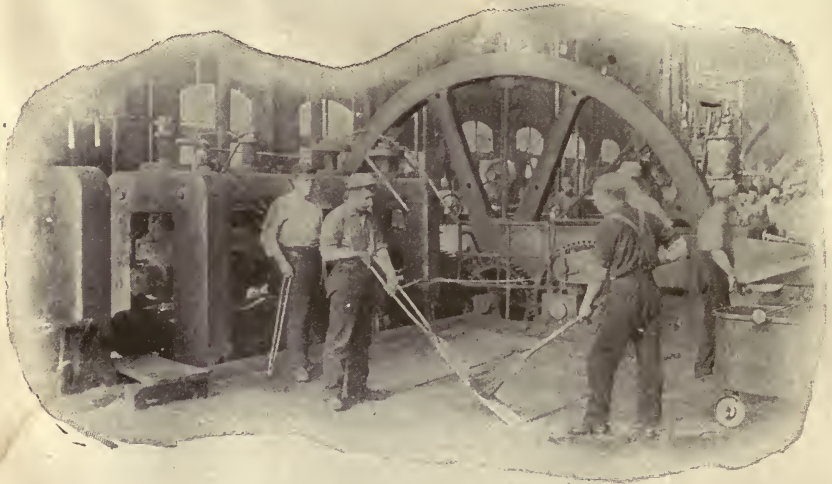
Ready for Rolling Long-Saw Plate.
